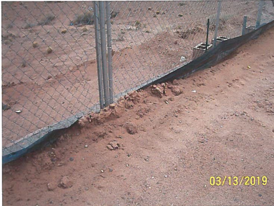
Grade higher than halfway up silt fence.
