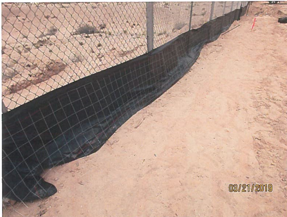
Silt fence not buried along western edge.
