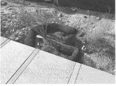
4. The area of land disturbance has been inactive for more than 14 calendar days and remains un-stabilized in violation of CGP Part 2.2.14. The site has remained unchanged since the last inspection (8/2/23).\
