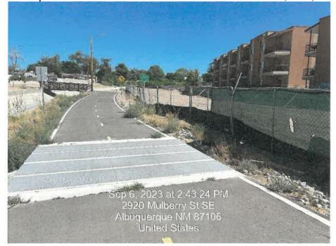
4. The area of land disturbance has been inactive for more than 14 calendar days and remains un-stabilized in violation of CGP Part 2.2.14. The site has remained unchanged since the inspection performed on 8/2/23.
