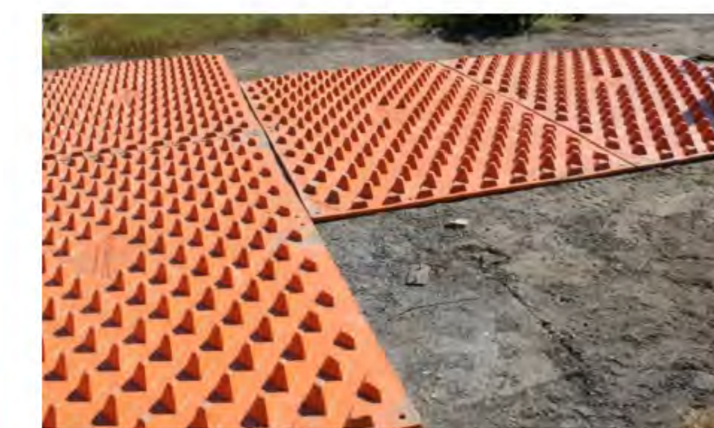
INSTALL FODS ACCORDING TO THE MANUFACTURER'S SPECIFICATIONS. FODS TRACKOUT CONTROL MATS CAN BE USED WITH A STABILIZED CE OR ALONE, AS LONG AS THEY CAN ACCOMMODATE THE TURNING MOVEMENTS OF THE LARGEST VEHICLES EXITING THE SITE.
