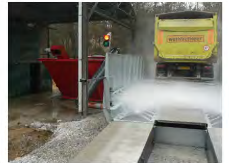
WHEEL WASH - PRESSURE WASHING DIRT OFF VEHICLE WHEELS CAN BE VERY EFFECTIVE. WHEEL WASH WASTEWATER IS PROCESS WATER, NOT STORMWATER. IT MUST BE DISCHARGED TO A SEPARATE ON-SITE TREATMENT SYSTEM THAT PREVENTS ITS RELEASE FROM THE SITE.
