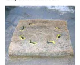
3. Position the mat. Place Inlet Filter on grate with the net side down, flush to the back edge and extending beyond the grate opening on the front and both sides. The zip ties attach Inlet Filter to the inlet grate cover WITHOUT LIFTING THE GRATE COVER.
