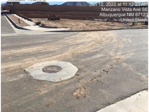
Washout also on Lobo Trout Ct. w/ no smaller washout containers at the houses to make washout of stucco and paint convenient to workers. (Violation Notification #1)
