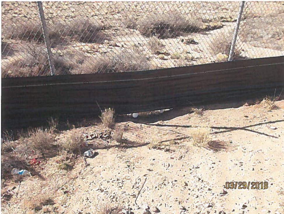
Silt fence not installed properly, it is not buried.
