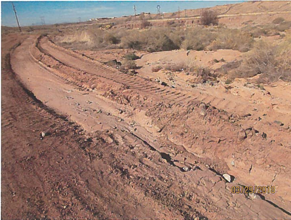
Undersized ponding area with uncompacted berm. Drainage bypassing stormwater quality pond.
