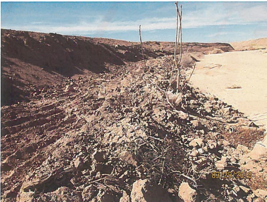
Loose soil in low-flow area of arroyo. Uncompacted berm
