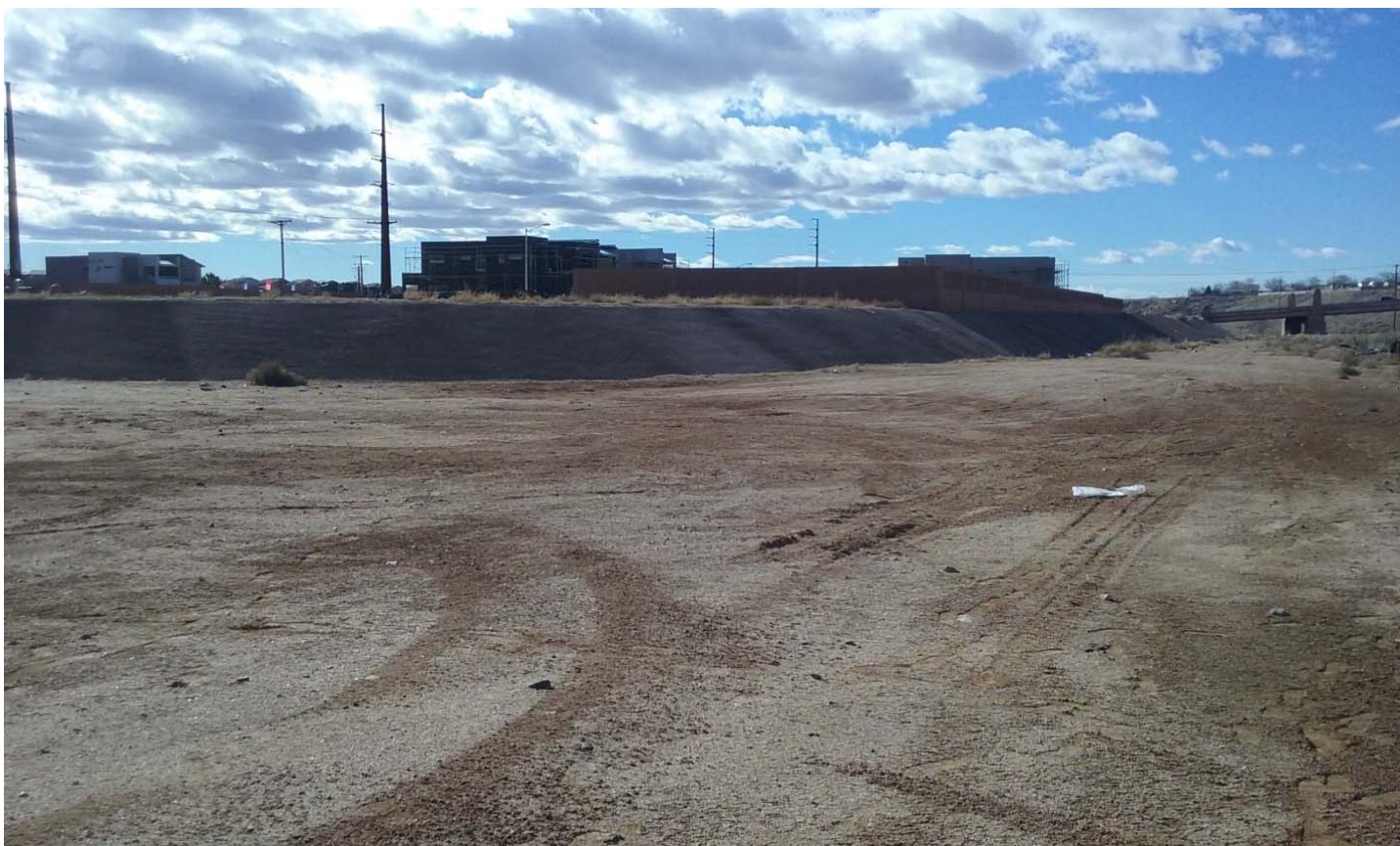
The Open Space west of Unit 3B was also filled to remove an ineffective flow area at Section 46 behind the newly constructed shotcrete bank protection.
