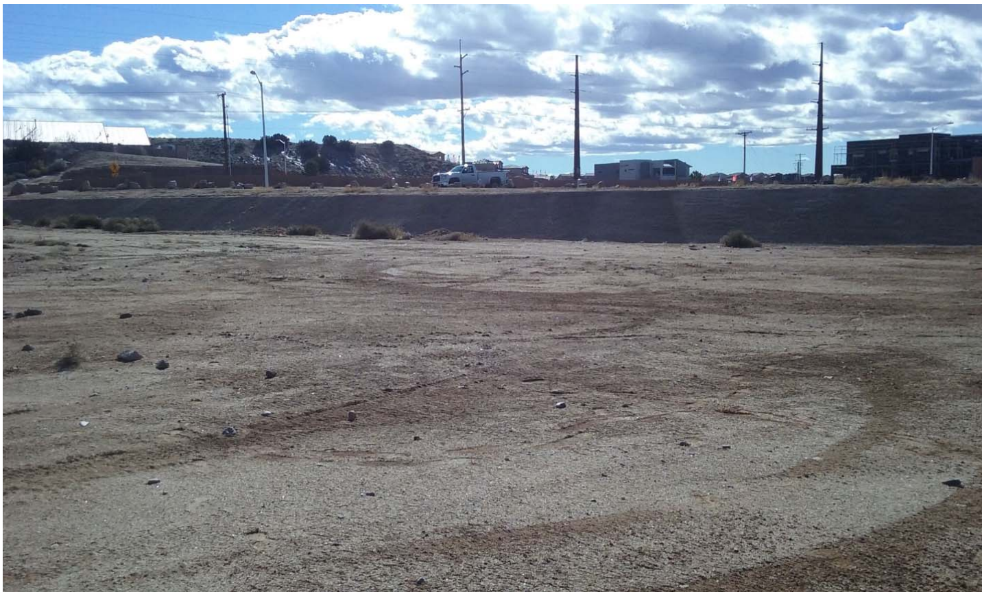
The Open Space west of Unit 3B was also filled to remove an ineffective flow area at Section 46 behind the newly constructed shotcrete bank protection.
