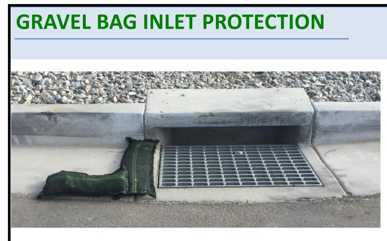
Inlet gravel bags are manufactured on site to fit in the gutter pan on the upstream side of the inlet. Filled with smooth rounded pea gravel. The ends are sealed with  $\frac{1}{2}$ " #12 hog rings. The gravel bags are connected together with the hogs to help create weight and stability.
