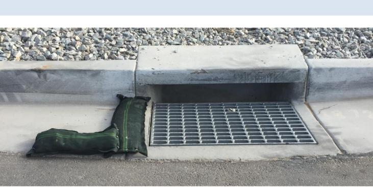
Inlet gravel bags are manufactured on site to fit in the gutter pan on the upstream side of the inlet. Filled with smooth rounded pea gravel. The ends are sealed with  $\frac{1}{2}$ " #12 hog rings. The gravel bags are connected together with the hogs to help create weight and stability.
