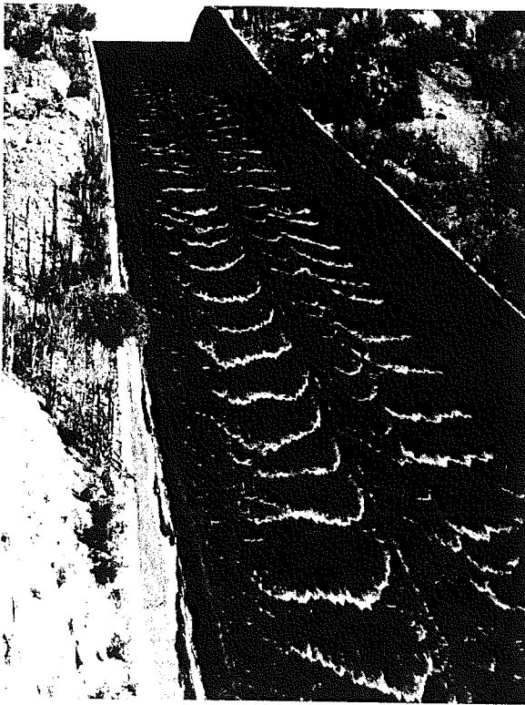
Figure 2-43. Unstable flow at shallow depth. H-686-55D
