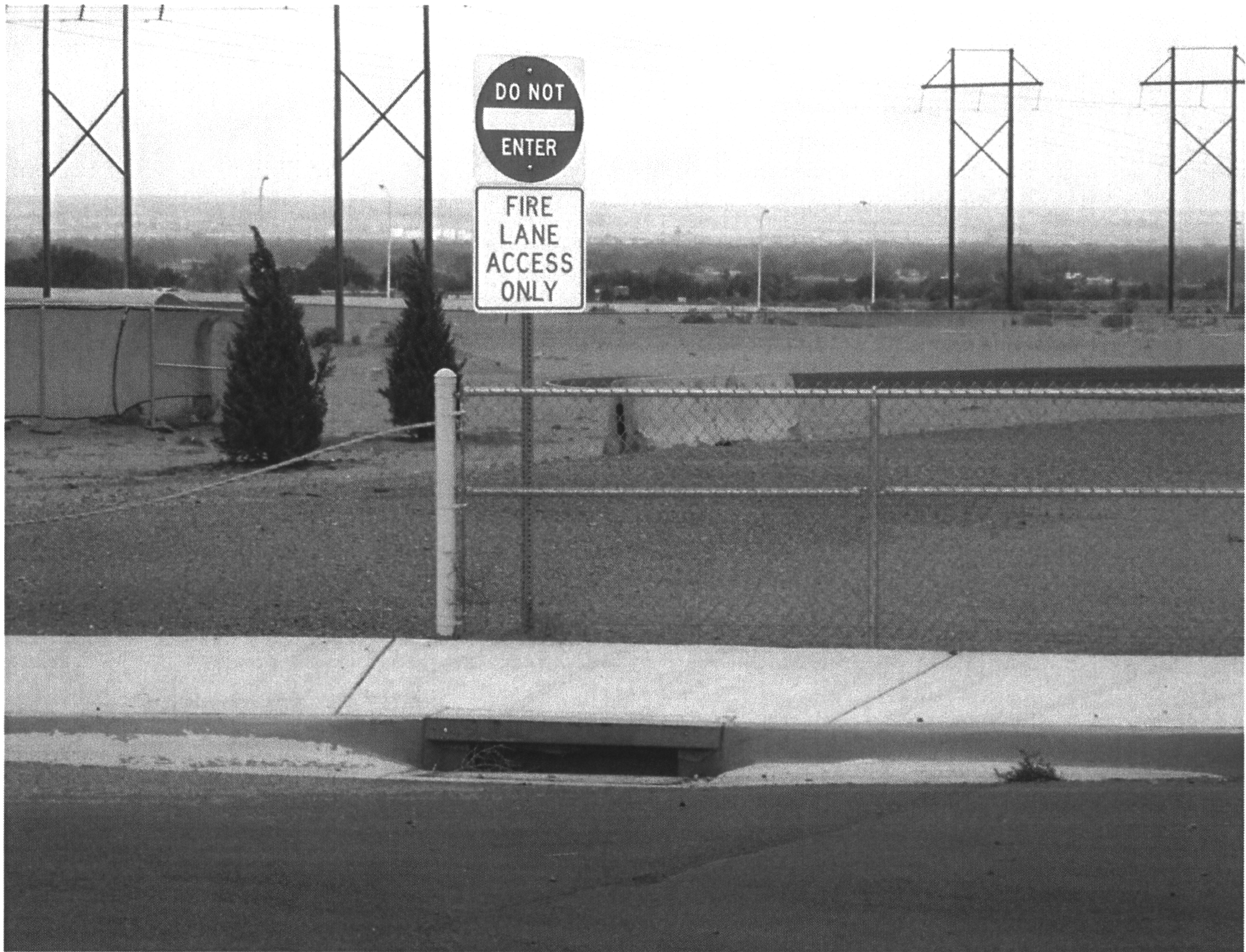
FIGURE 1: Single C storm inlet downstream of portable site at east end of bus loop.
