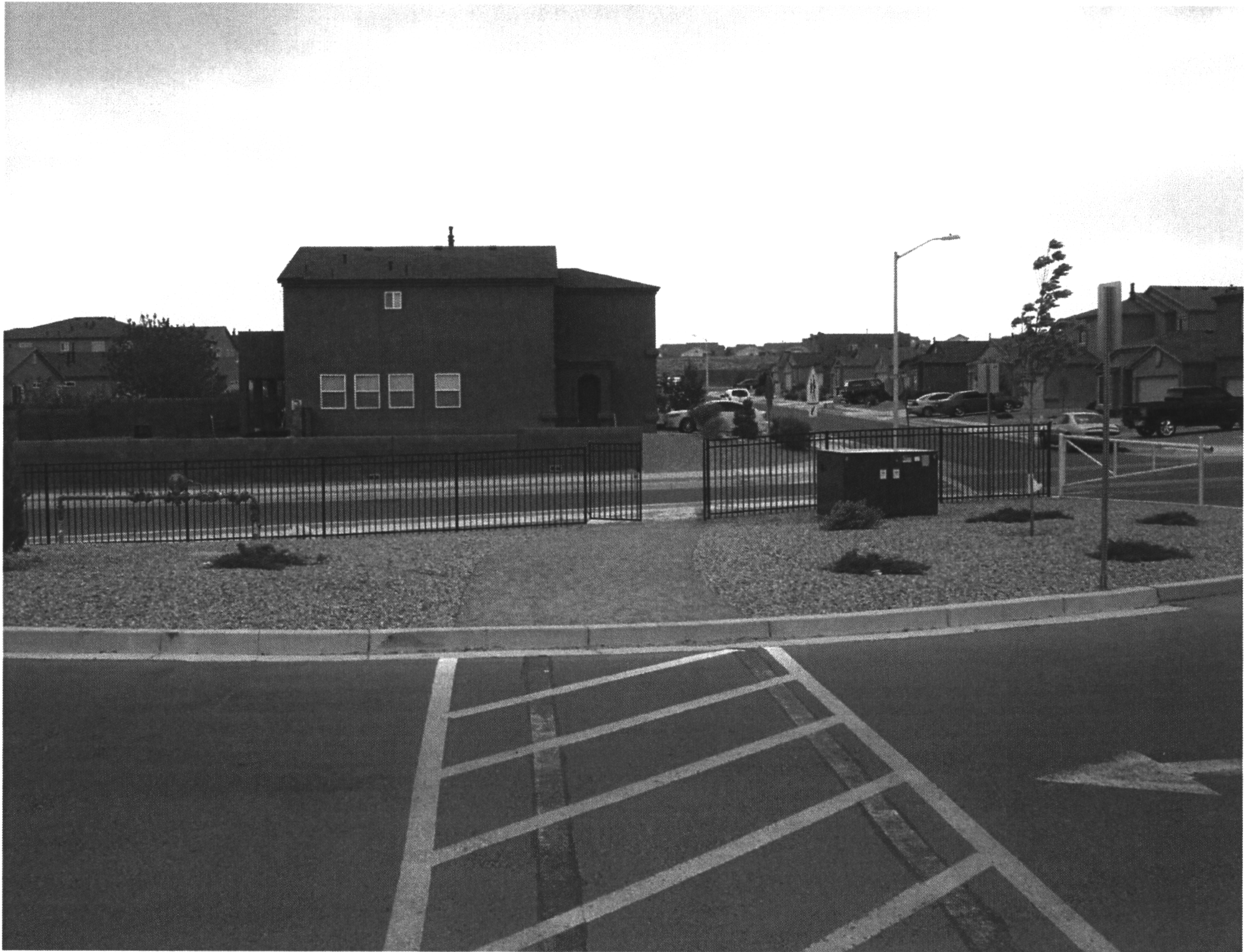
FIGURE 6: Continuation of crusher fines path; crosswalk must remain to maintain access to this walk. Walk is not ADA.
