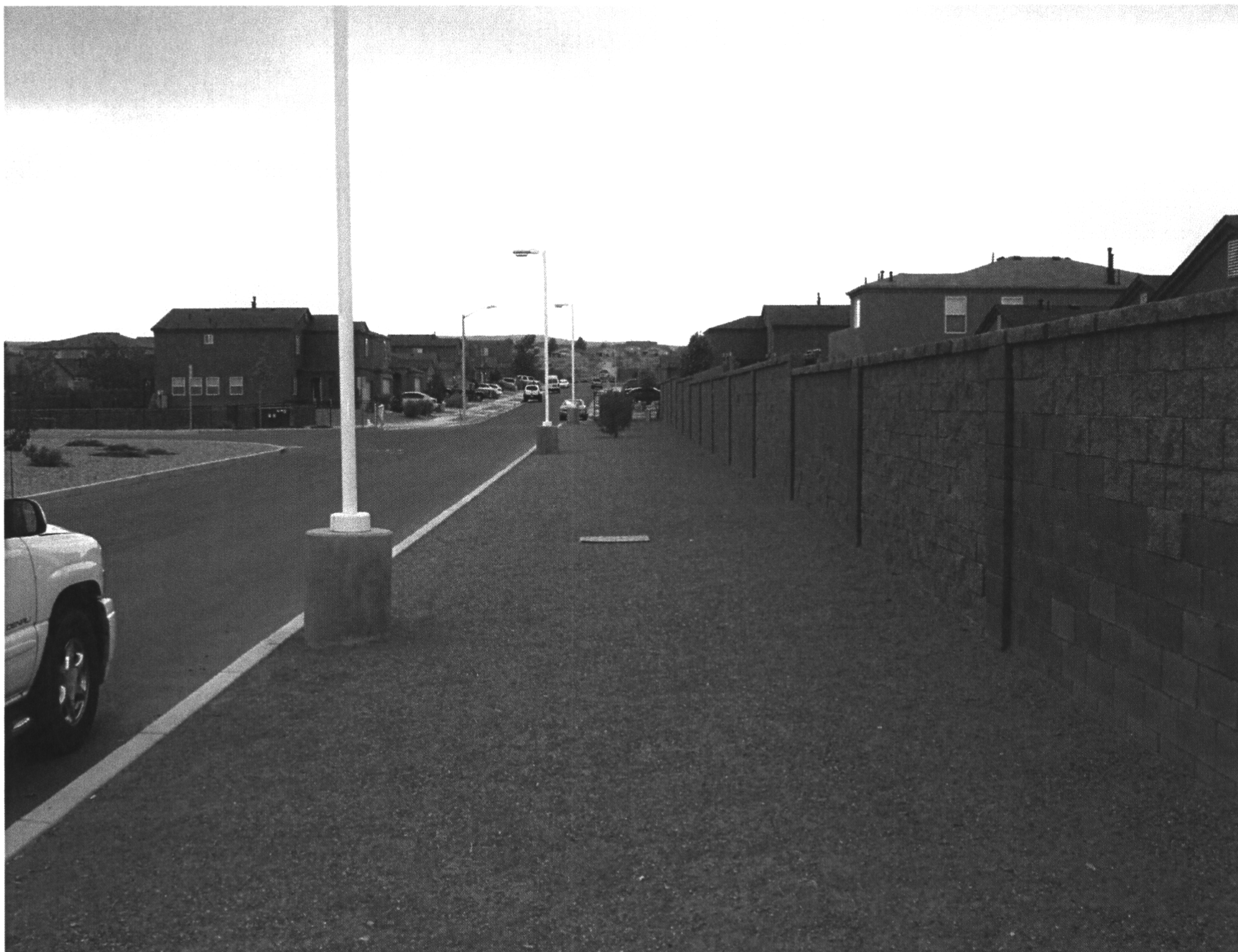
FIGURE 2: North edge of school site where surface is stabilized with minimal landscaping and crusher fines ground cover.
