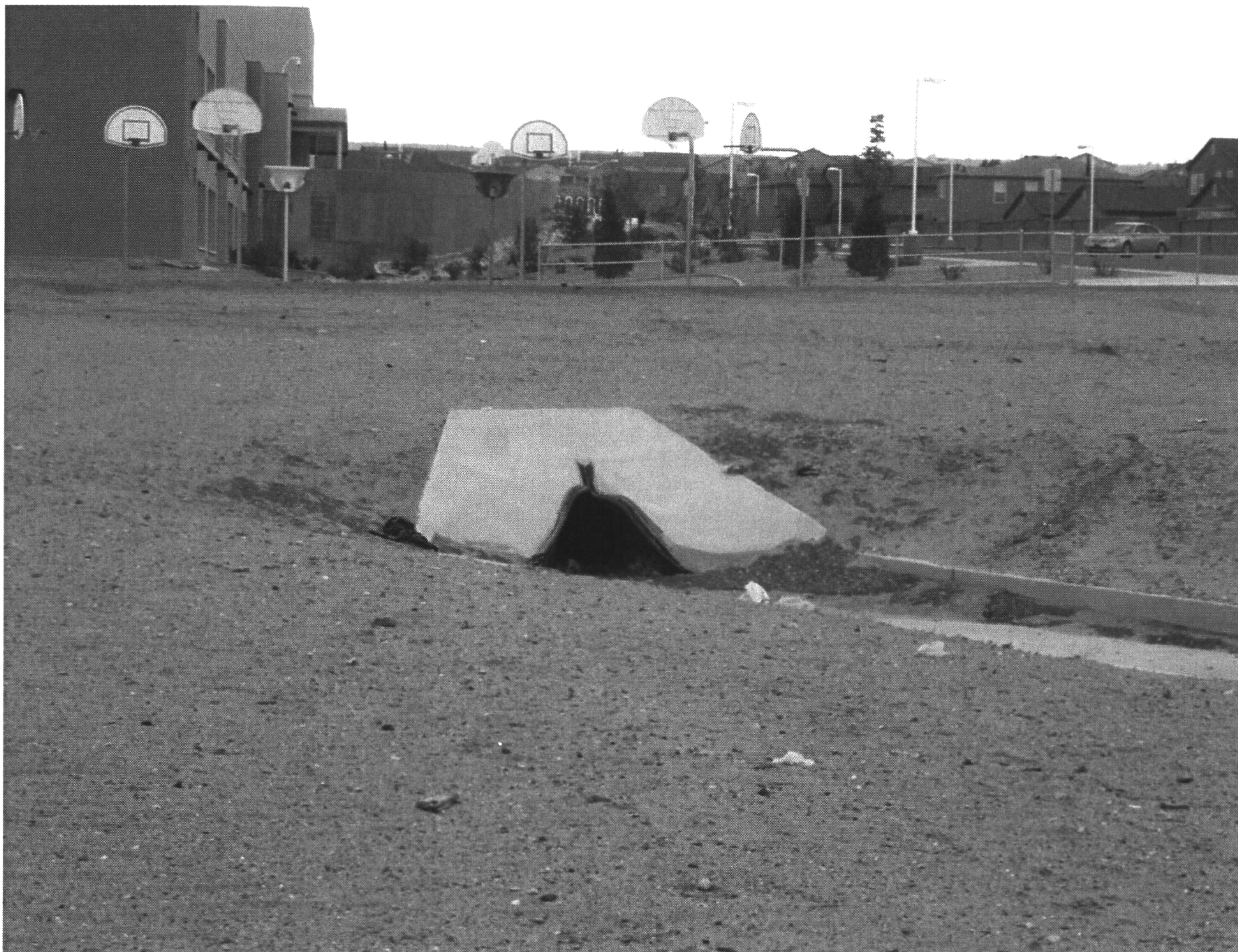
FIGURE 7: Downstream storm drain outlet. This appears to be the outfall for the Single C Storm Inlet depicted in Figure 1.
