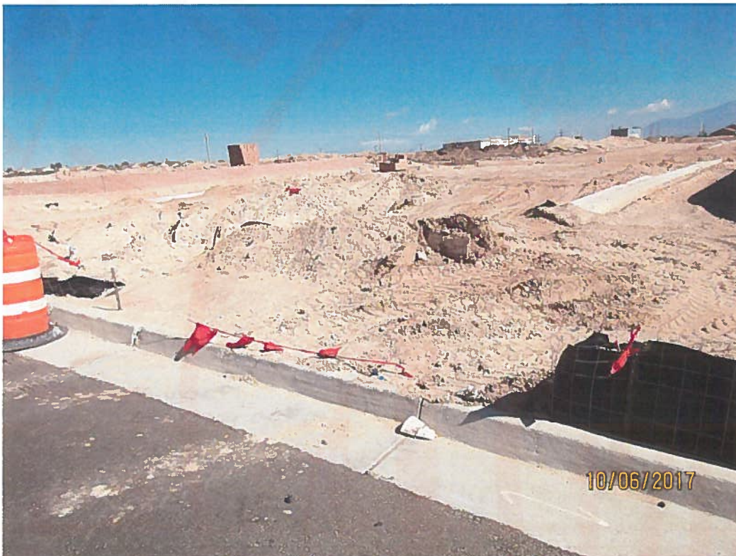
Site exit without a track-out pad. Silt fence missing.
