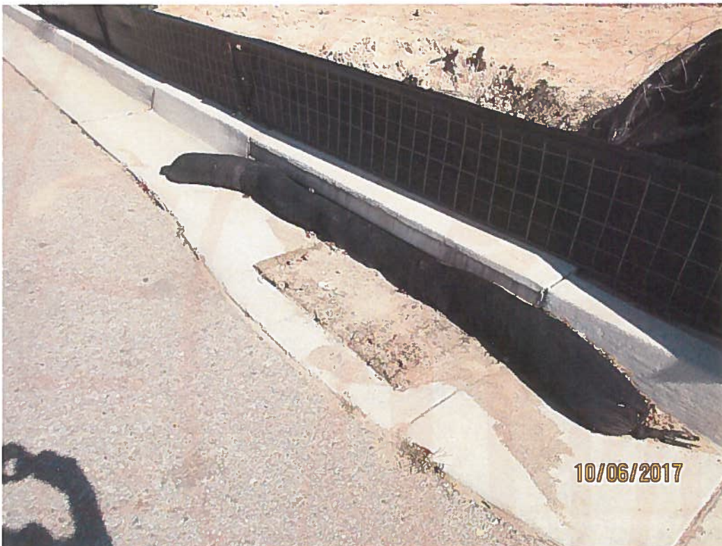
Inlet protection requires maintenance.
