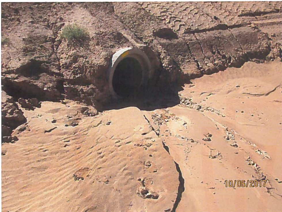
Pond outfall without a sediment BMP. Sediment entered the City's drainage system.
