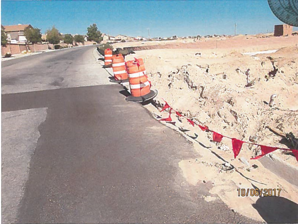
Dirt pile along Blake Rd. No sediment BMP.
