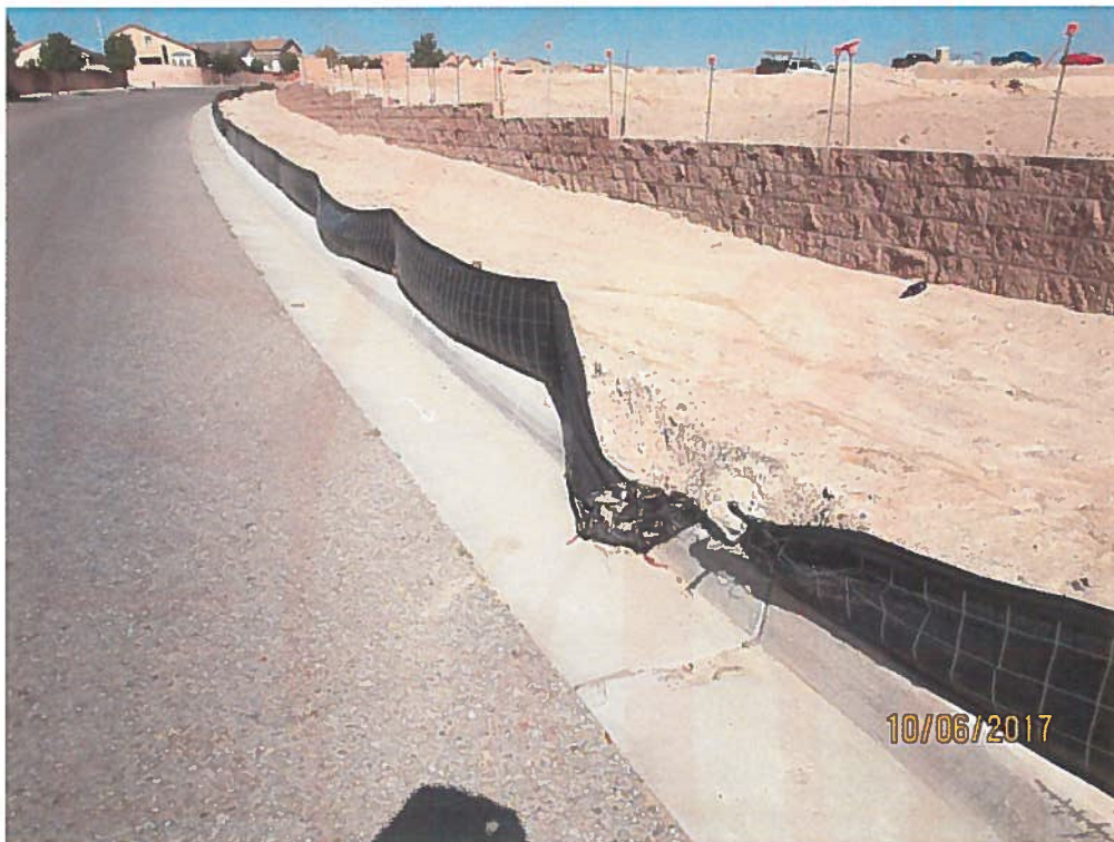
Silt fence requires maintenance.
