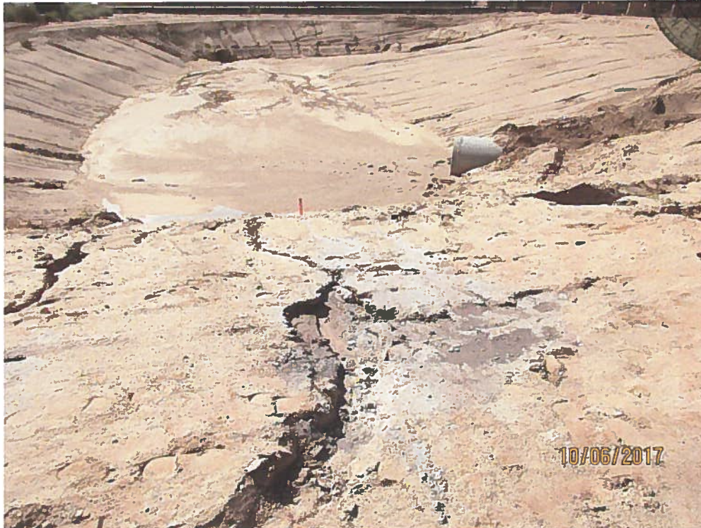
Wash-out draining into pond that outfalls to City's drainage system.
