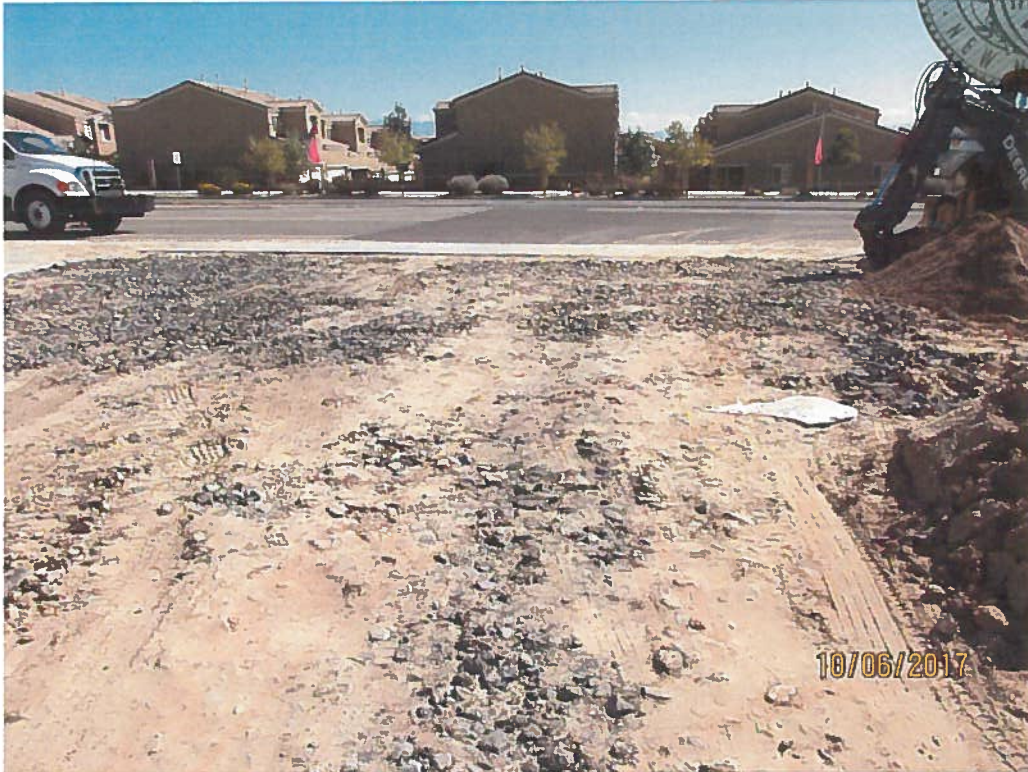
Track-out pad requires maintenance.
