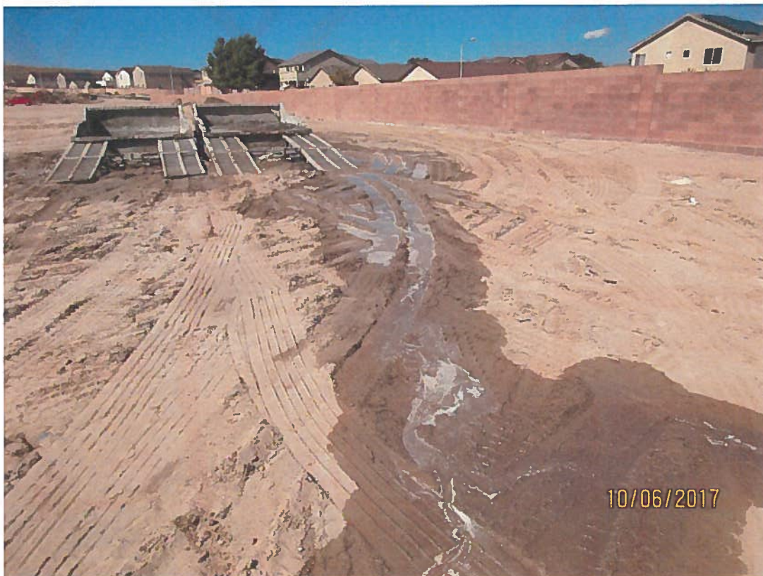
Wash-out facility full, overflowing and draining away.
