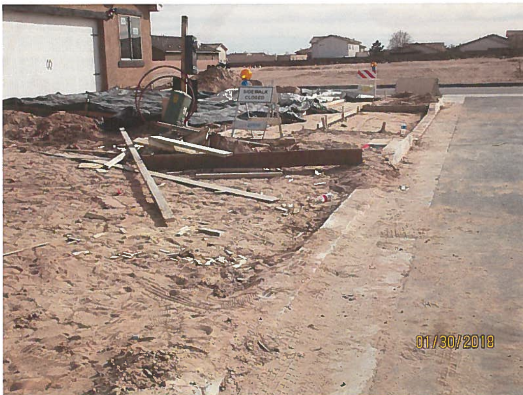
Sediment in gutter and street. Inadequate sediment BMP on lot.
