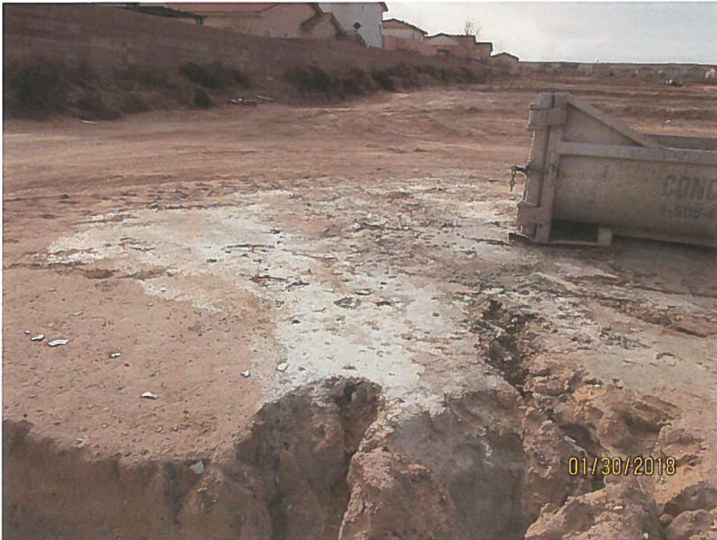
Wash-out not in wash-out facility.
