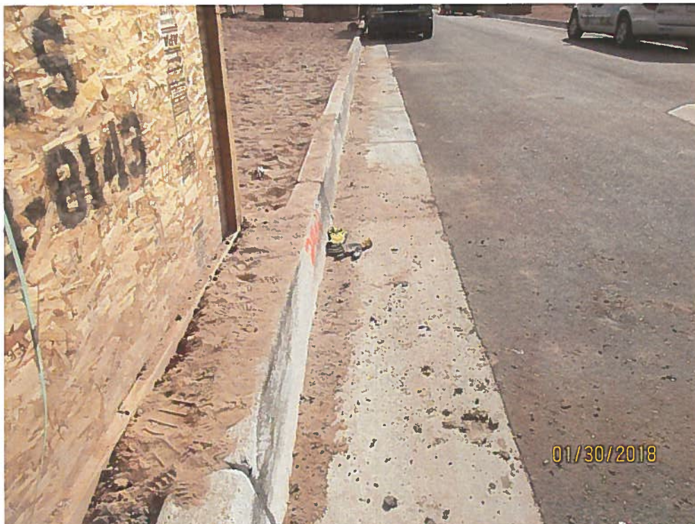
Sediment and trash in gutter. Inadequate BMP on lot(s).
