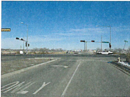
NB Prince St. at Rio Bravo Blvd.
