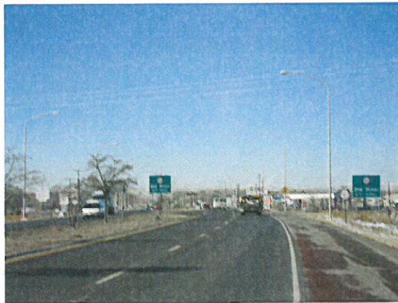
Westbound Rio Bravo Boulevard east of Second Street
