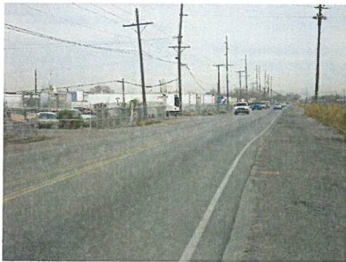
Second Street north Rio Bravo Blvd. looking northbound
