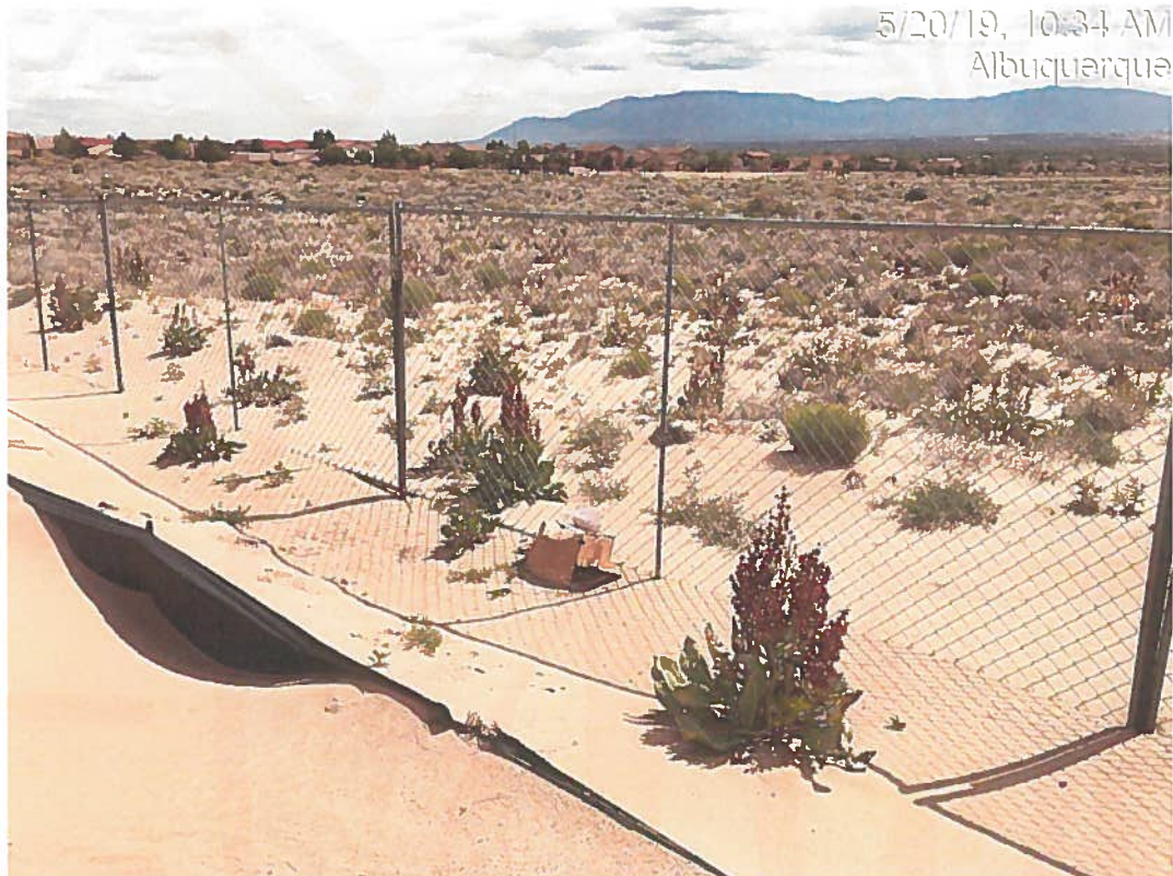
Sediment from the construction site has blown offsite. Silt fence is full.
