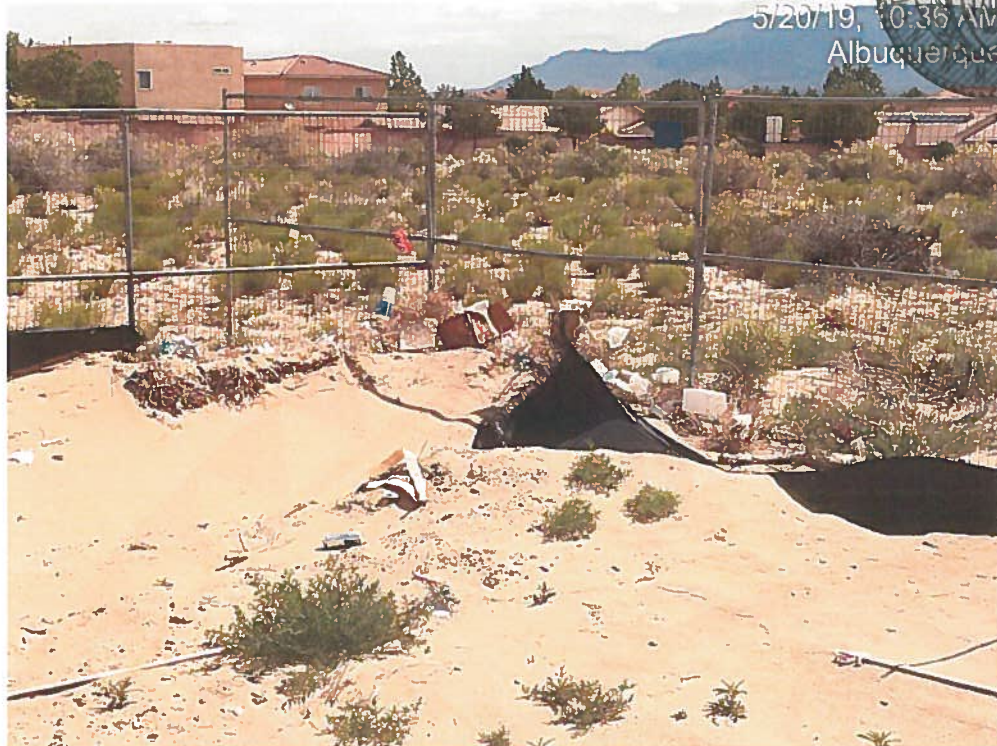
Silt fence requires maintenance and construction and domestic waste not in an acceptable container.
