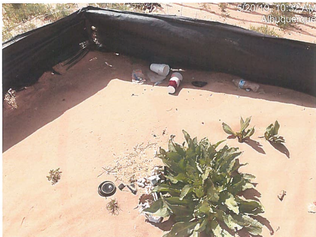
Domestic waste not in an acceptable container. Silt fence is torn.
