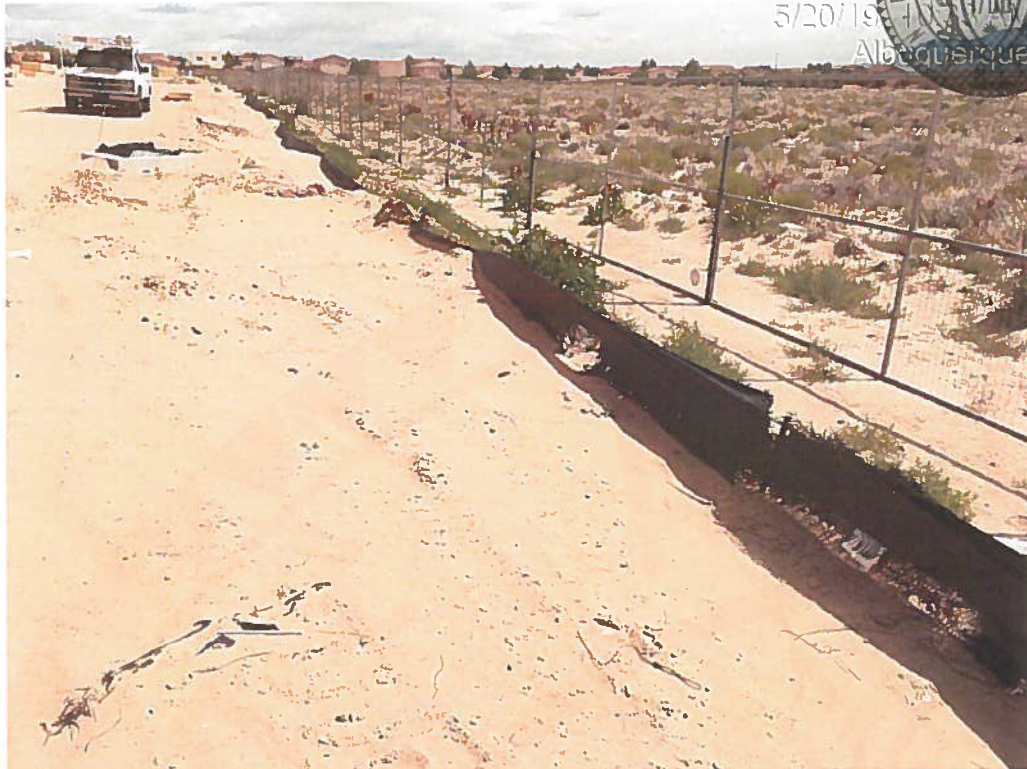
Silt fence is torn.
