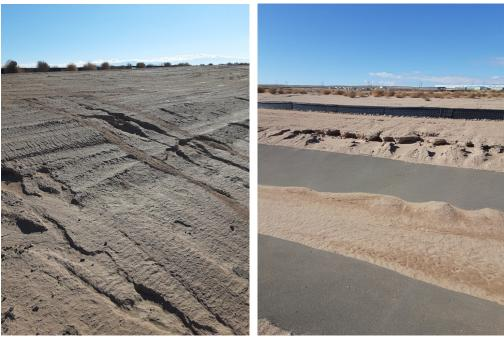
4. It also appears that the pond was not built per the construction plans. There was not berm built around the pond, the emergency spillway does not appear to be built, and section A-
