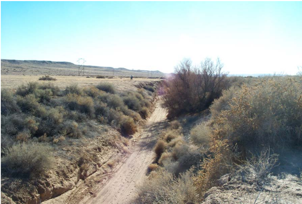
Plate B.2. View downstream of Tijeras Arroyo in the vicinity of the proposed bridge crossing.
