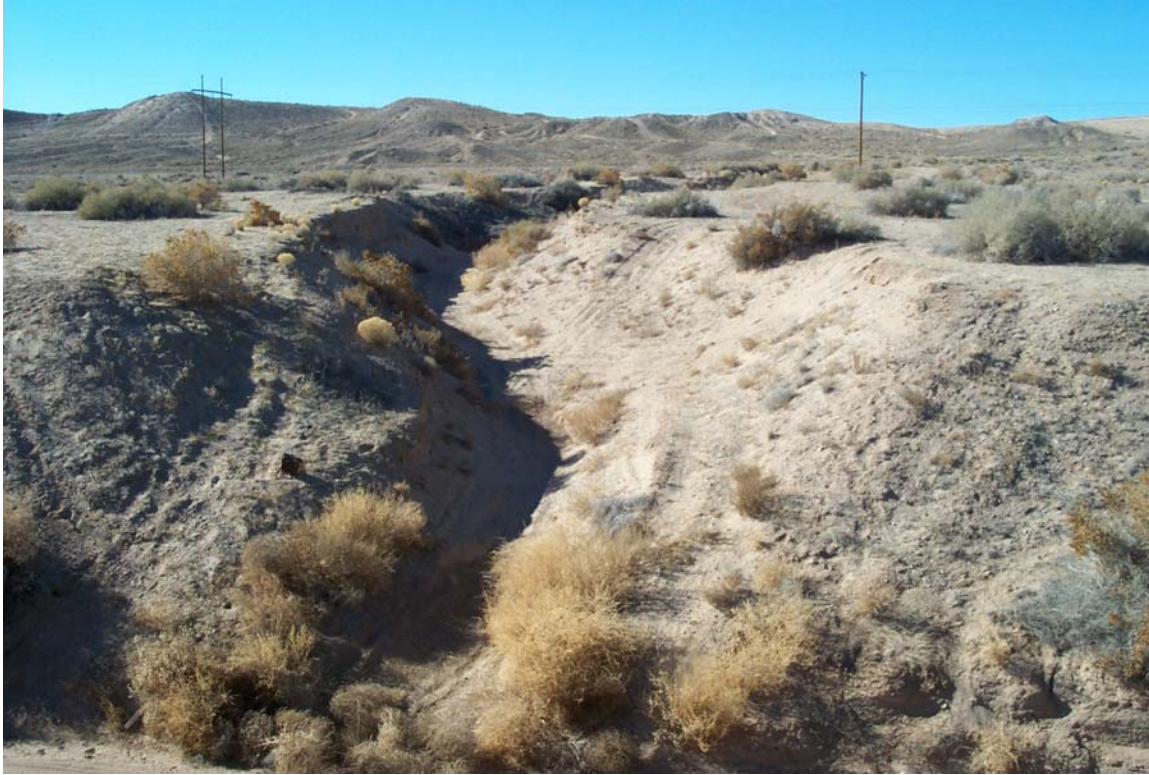
Plate B.5. View across Tijeras Arroyo of incised tributary located on the right bank about 30 feet downstream of the proposed bridge.
