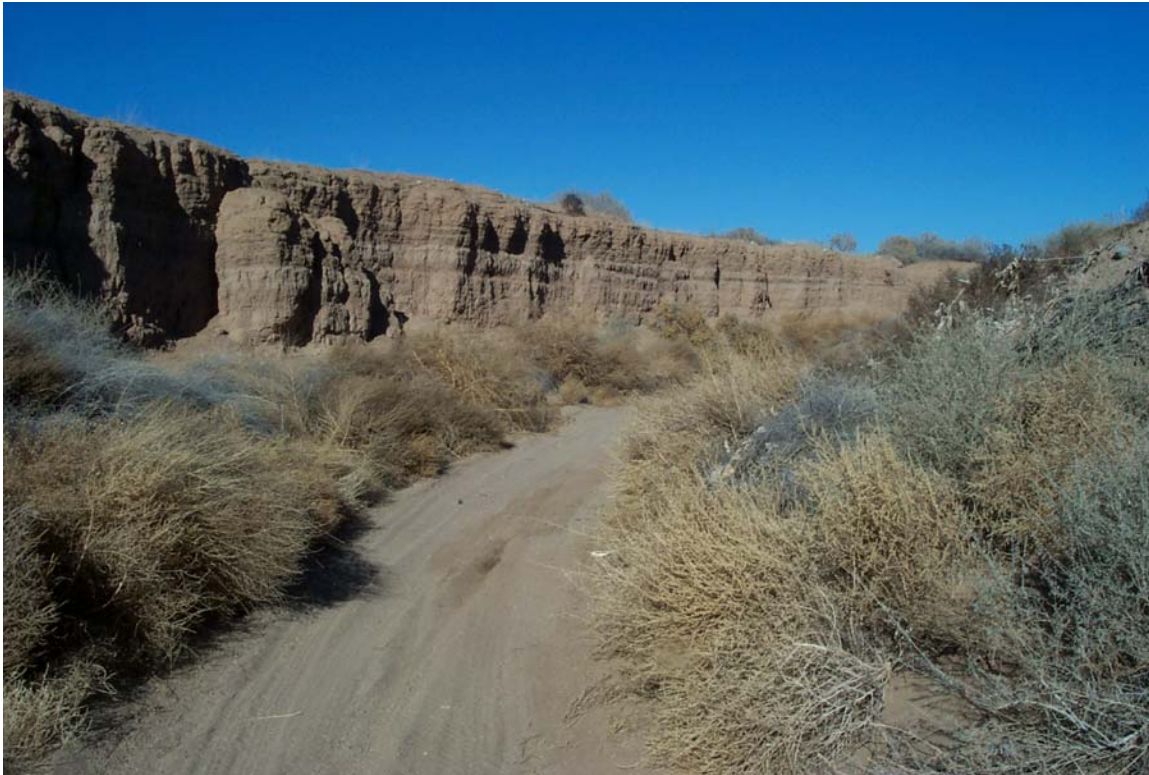
Plate B.1. View looking downstream of Tijeras Arroyo about 200 feet upstream of the proposed bridge.
