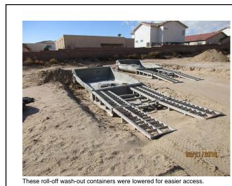
1. Designated wash-out areas shall be provided for any concrete, stucco, mortar, or paint operations. Wash-outs should be as far away as possible from waters of the U.S., stormwater
