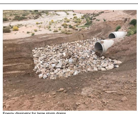
Energy dissipator for large storm drains
