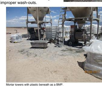
5. Mortar towers shall have a plastic liner beneath them to prevent the wet mortar from contacting the soil. If wet stucco or mortar contacts the ground due to mixing, it would be a compliance issue.
