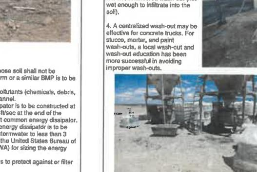
5. Mortar towers shall have a plastic liner beneath them to prevent the wet mortar from contacting the soil, if wet stucco or mortar contacts the ground due to mixing, it would be a compliance issue.
