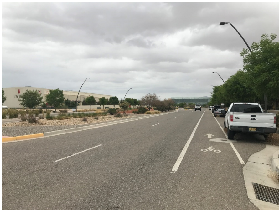
Figure 5. Southbound University Boulevard at Site
