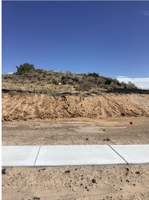
Site Walk Deficiency Photos - perimeter silt fence
